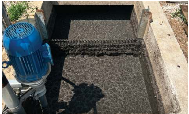
ADDITIONAL SCREENING FOR HOG PIT
